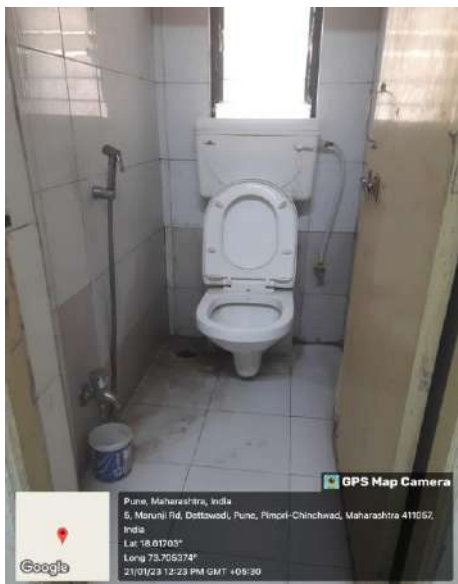
Washroom for Divyanjan students
