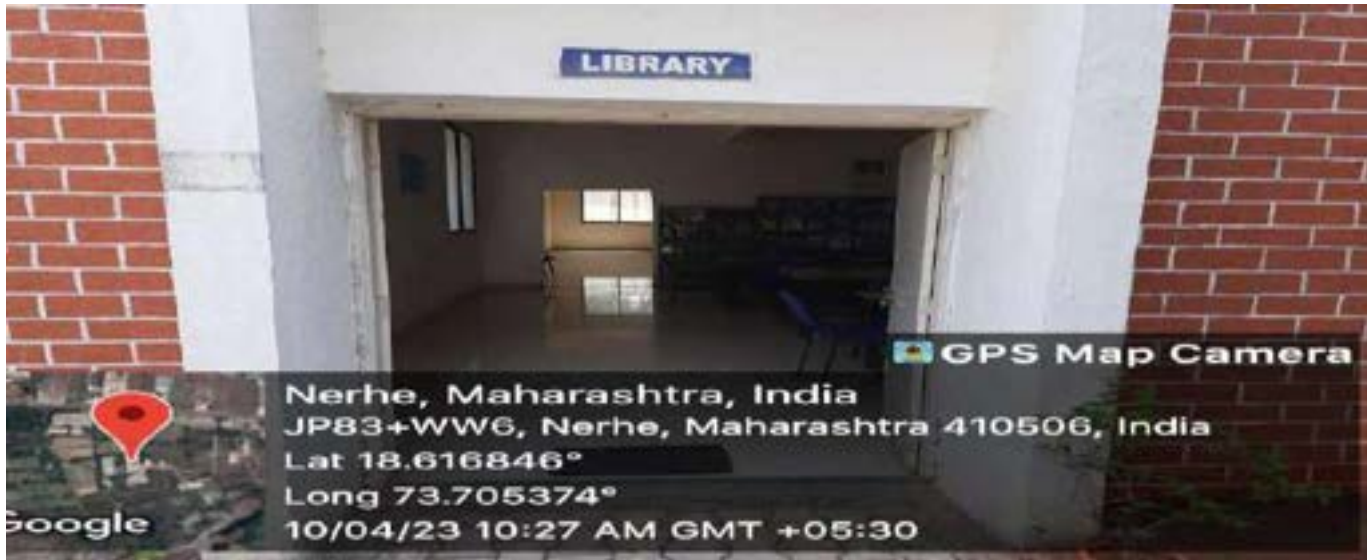
Library Entrance Gate
